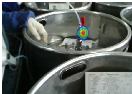
Gas pipeline leakage
