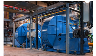
Noise and vibration
